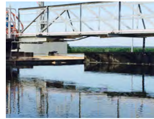
Treatment Facilities, Pumps, Lift Stations and Sewers
